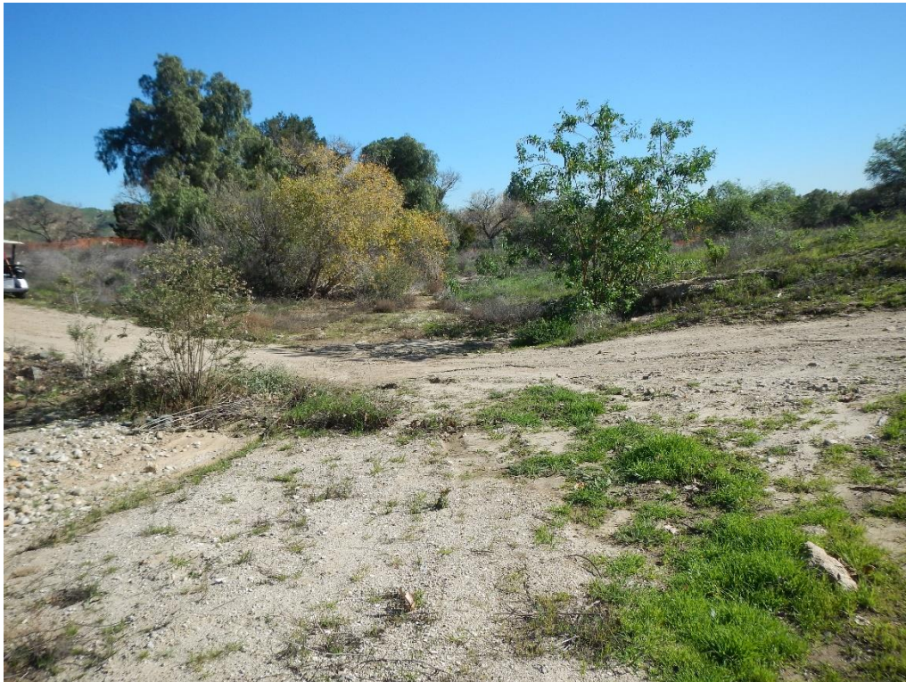
Photograph 8: Looking downstream at Aliso Canyon and the existing maintenance trail at the proposed span bridge location.
