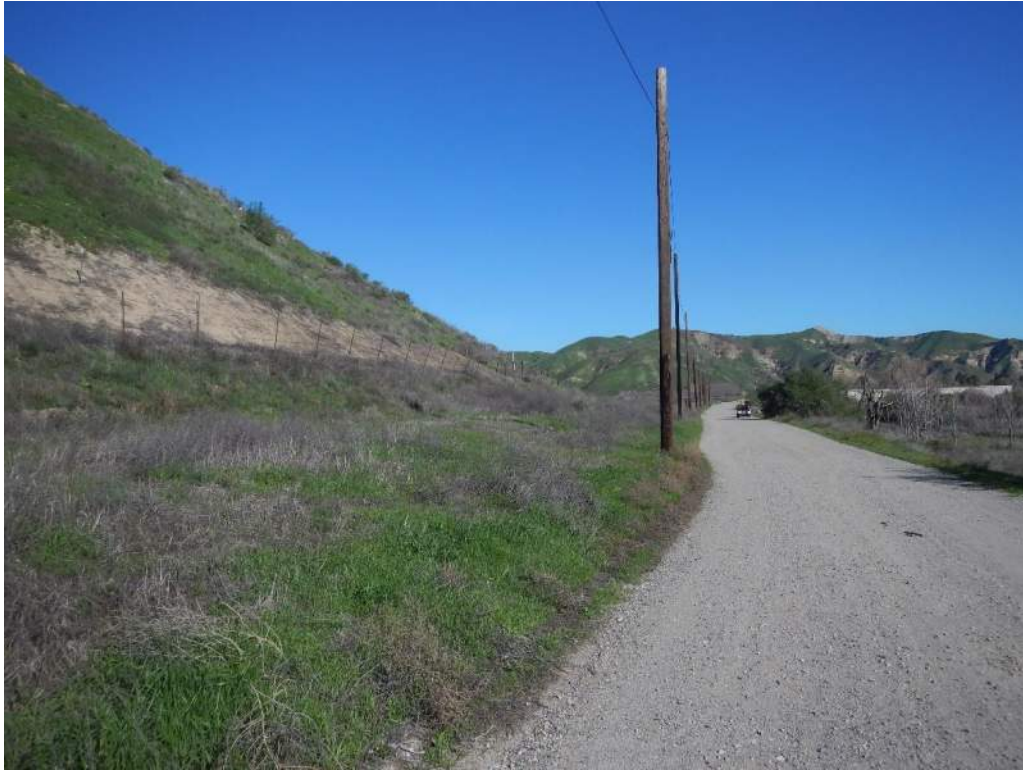
Photograph 5: View of existing access road and Alternative 1 alignment located to the west of the Green River Golf Course, facing north.
