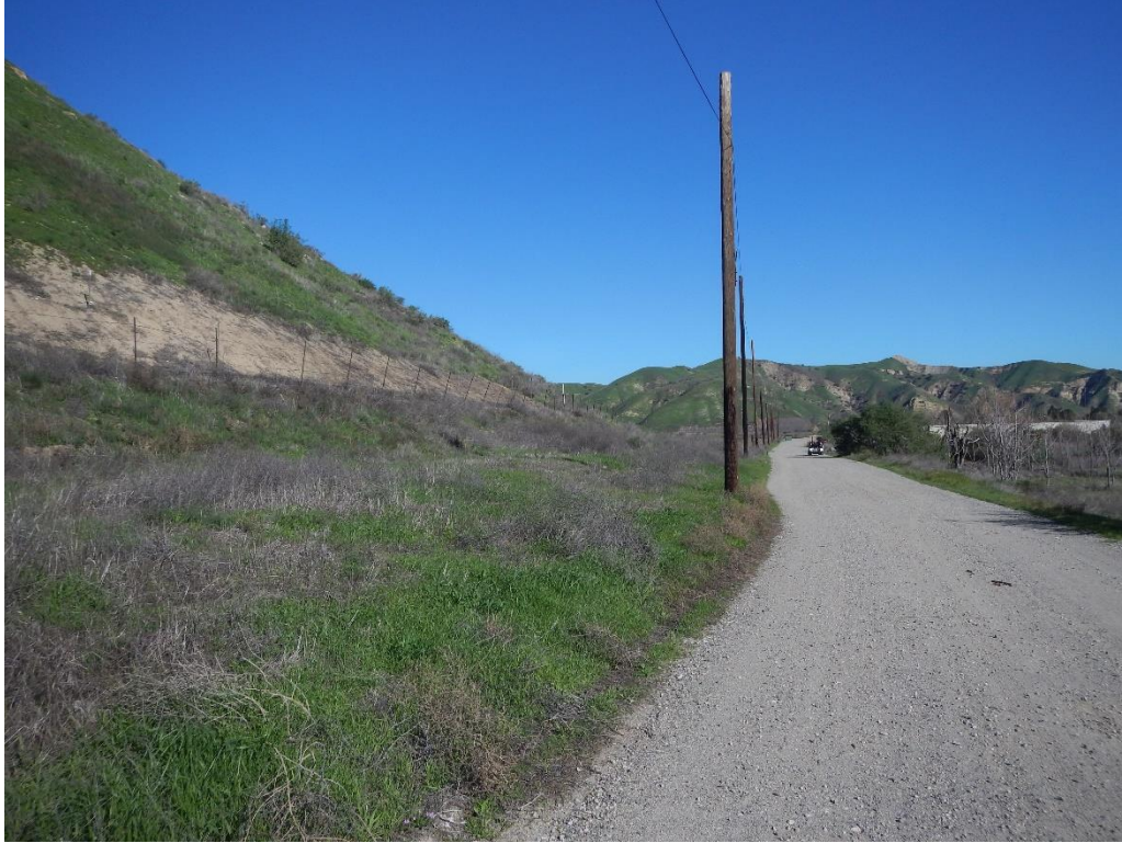
Photograph 5: View of existing access road and Alternative 1 alignment located to the west of the Green River Golf Course, facing north.
