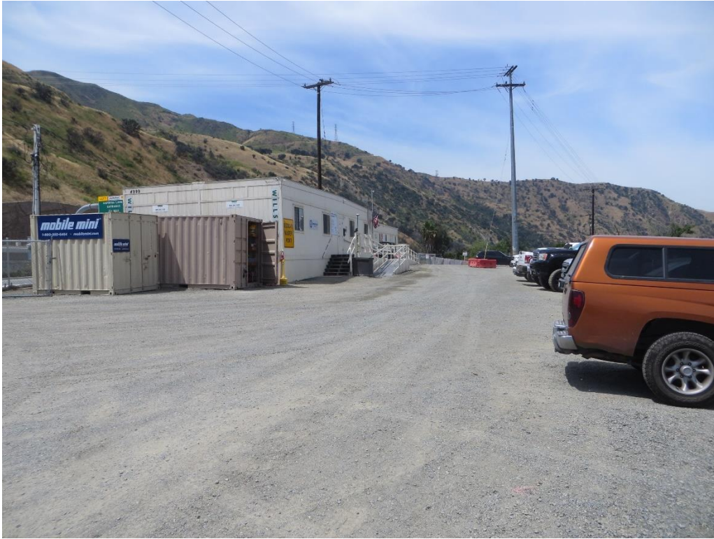
Photograph 17: View of existing structures, parking lot, and staging area located along Green River Road, facing southwest.
