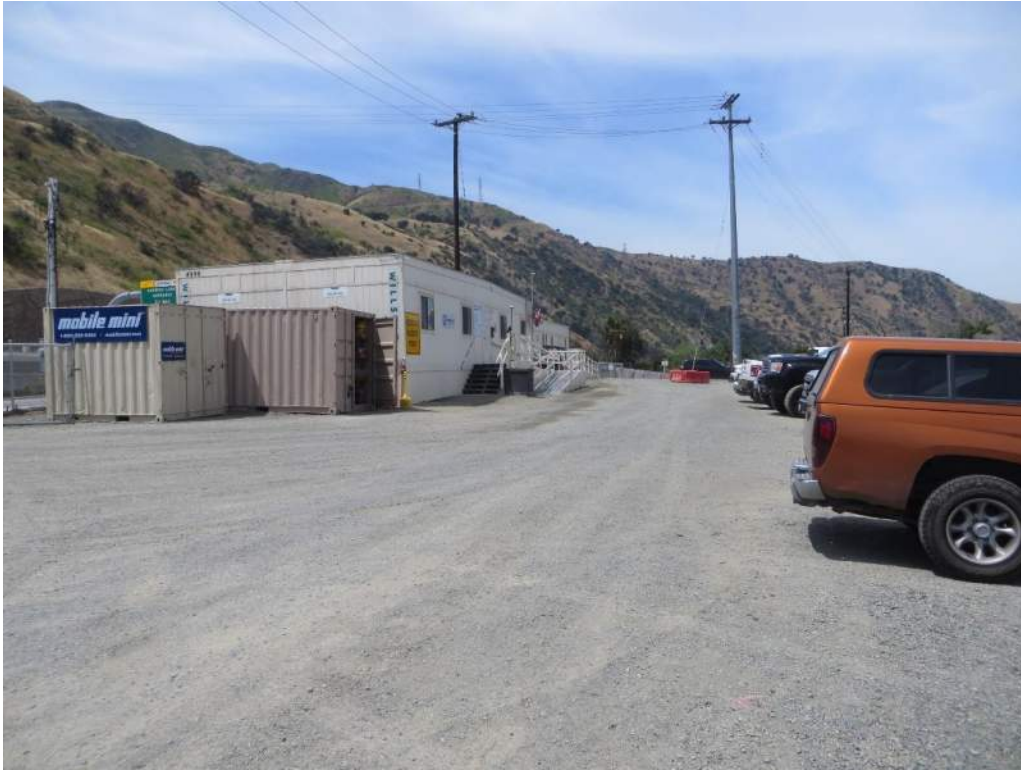
Photograph 17: View of existing structures, parking lot, and staging area located along Green River Road, facing southwest.
